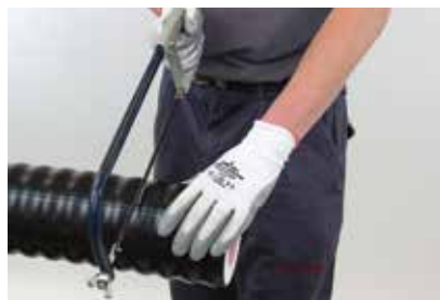
(2) Cut the casing pipe with a saw.
