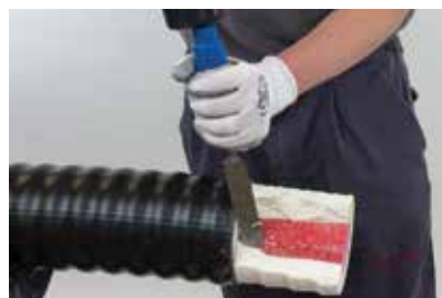
(5) Cut back and remove the insulation along the length (see table for dimensions L).
