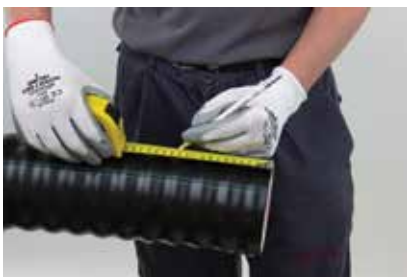
(1) Mark the distance plus 10mm from the end of the pipe.
