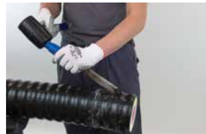
(3) Split the casing pipe with a knife or chisel. Note: Ensure you don't damage the service pipe.
