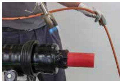
(8) Fit the Heat-Shrink End Cap (see section 5.4.1).
