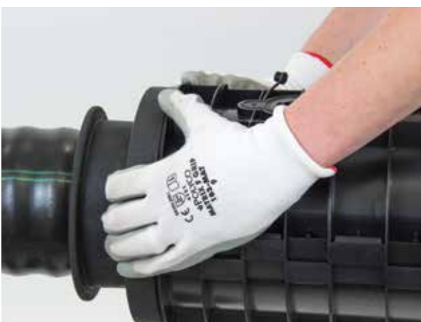
(5) Making sure that the sealing areas are clean and all catches have securely clicked together, pull the sealing rings over the ends of the two shell halves.
