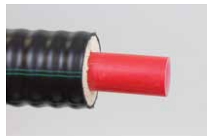
(6) Clear off remaining insulation from exposed pipe ends.
