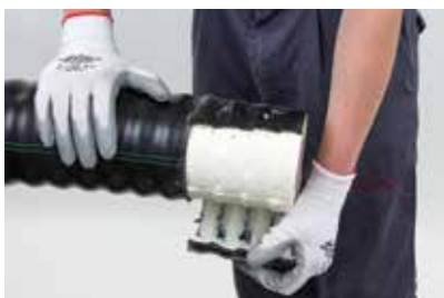
(4) Peel off the casing.
