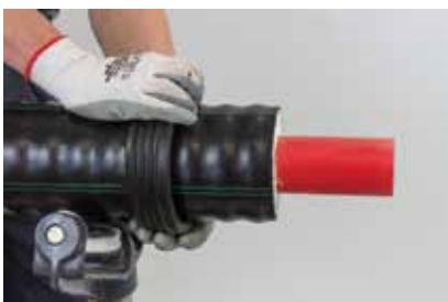
(7) Install the wall sealing ring.
