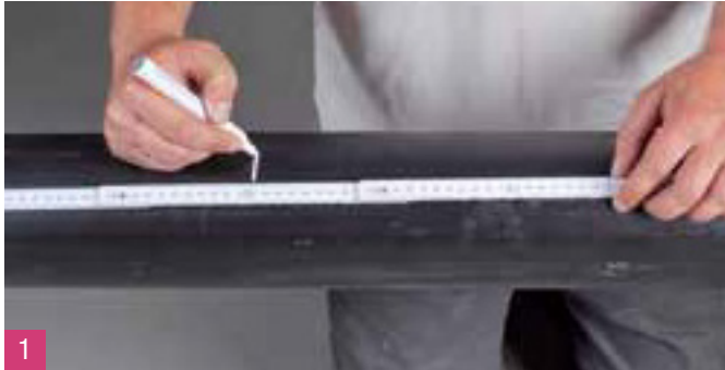
1 Measure the pipe length and mark on the casing pipe.
