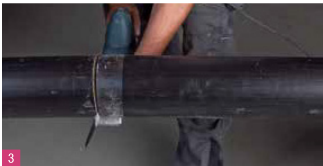
3 Cut the pipe with a customary handsaw with a saw blade for plastic along the cutting line.
