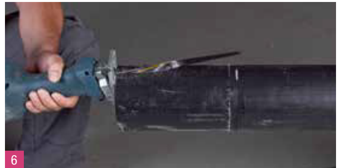
6 Slit the casing up to the PUR-insulation layer with a customary handsaw for plastic.
