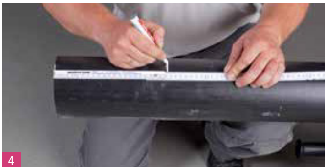
4 Mark the skinning length of 22.5 cm from the pipe end on the casing pipe.
