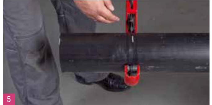
5 Cut the casing pipe with the pipe cutter up to the PUR-insulation layer around the whole pipe.
