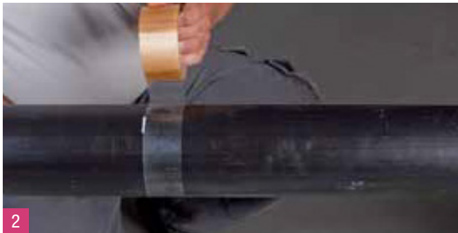
2 Mark the cutting line with an adhesive tape around the pipe.
